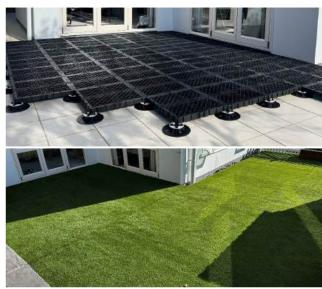
The Nuragrid system is a versatile and innovative solution for raised flooring projects. Its combination of durability and ease of installation makes it an ideal choice for both residential and commercial applications.
